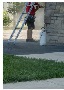
Tucking pointing being completed
